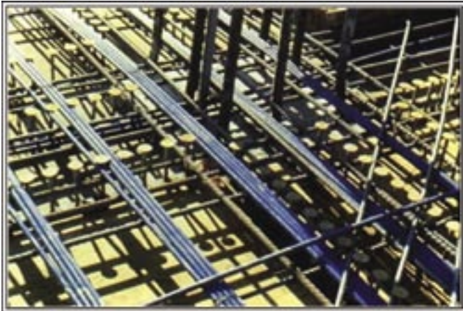
Fig. 2: This form of shear reinforcement is easy to install, without congestion or formwork interruption 5
