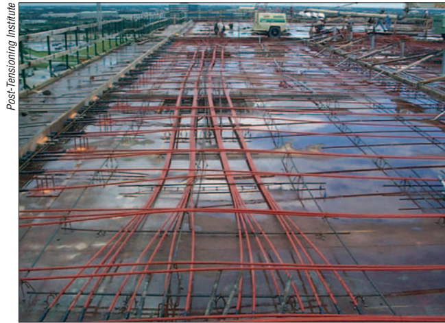
Figure 6: Banded tendons follow column lines with transverse tendons spaced uniformly.
